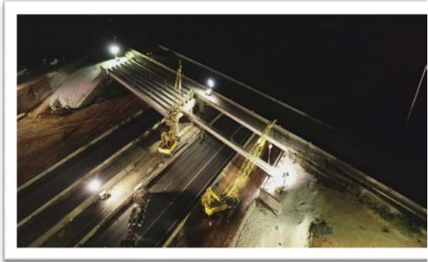
Figure 7 Exit 22 bridge beam being set in June 2019 (Photo: Edward Erb, CDM Smith)
